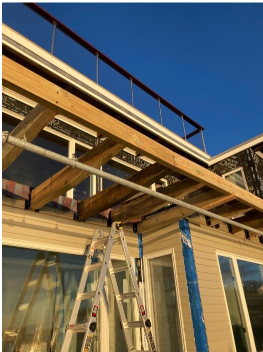
Framing underway for the second-floor deck
