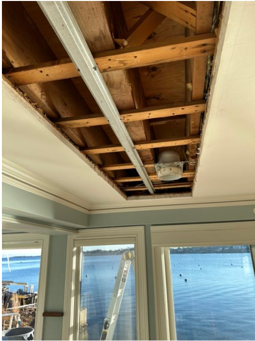
Opening a section of the first-floor ceiling to remove and replace rotten segments of support beams for the second floor deck.
