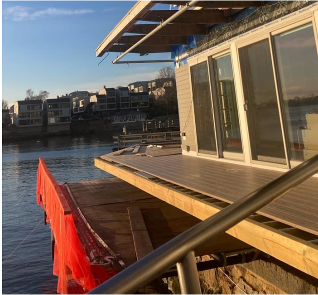
Figure 1 Current state of the first floor deck, waiting for the steel
