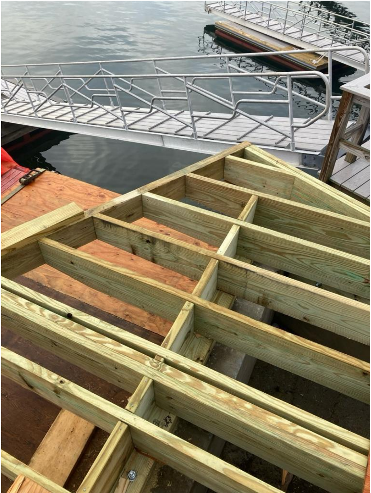
Figure 1 New framing of first floor South East Corner
