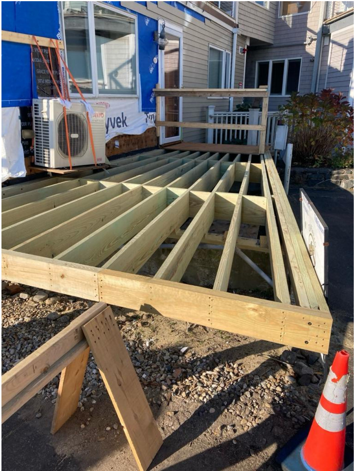
Figure 4 Reframed 1st floor North deck
