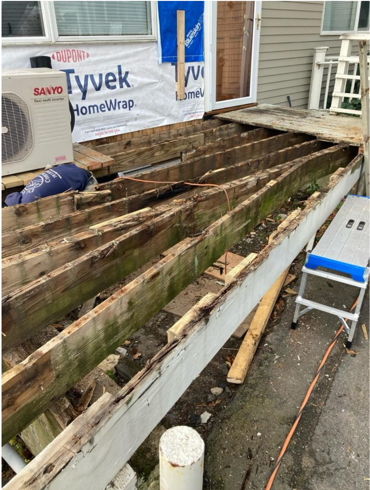
Figure 3 State of the 1st floor North Deck once decking was removed
