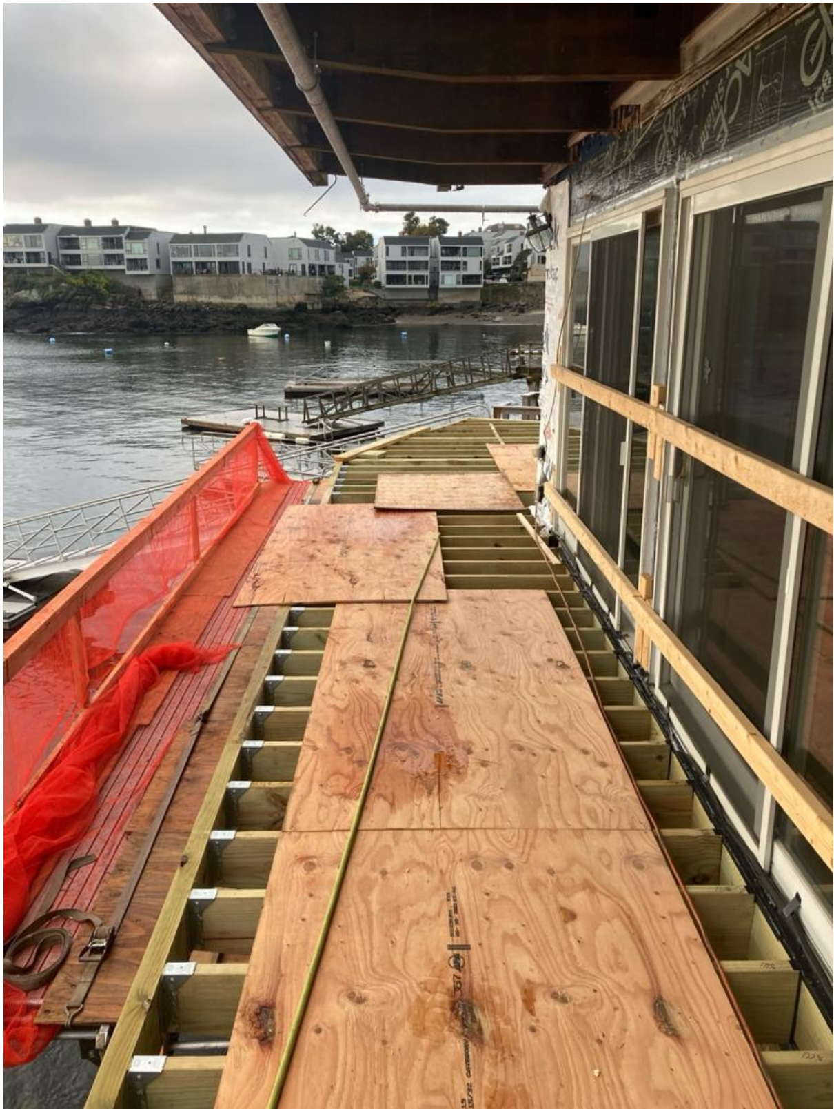
Figure 2 New framing of the 1st floor East Deck
