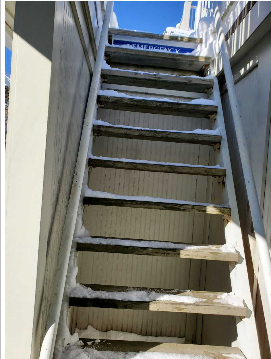
Emergency egress from upper Building A
