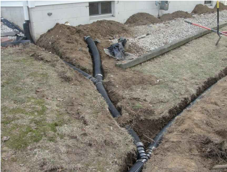
TYPICAL DOWNSPOUT/ROOF DRAIN SYSTEM NOT TO SCALE
